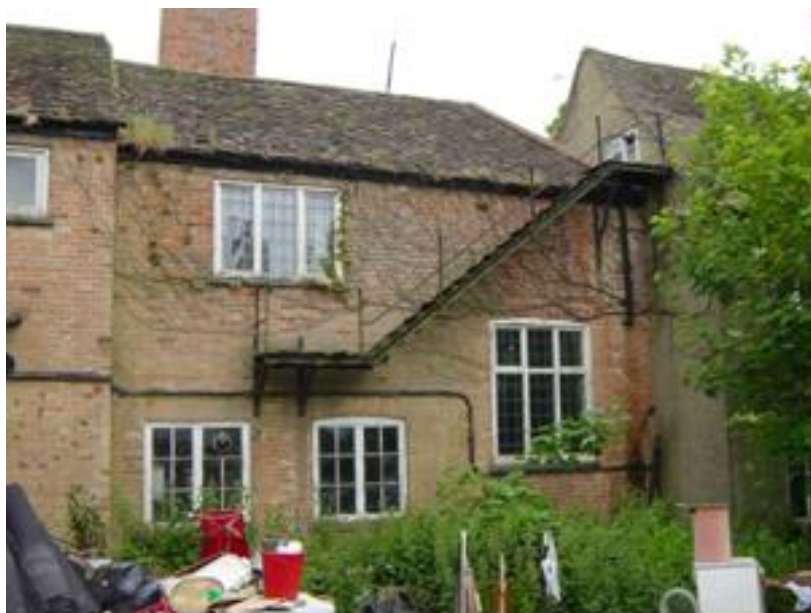
Part of the North face of the Hall from the courtyard, (Spring) – note the termination of the fire-escape!
